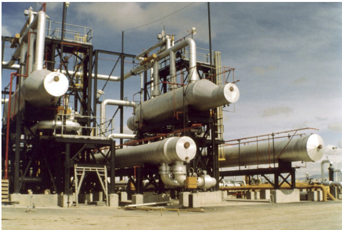
Fig. 20.12 Preheaters and evaporators: lower row (L-R) – HPH and LTH; upper row (L-R) – HPE and LPE [WWW].
