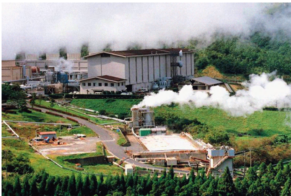
Fig. 14.11 District hot water heating facility at Hatchobaru. Direct-contact water heater is seen in the foreground, adjacent to settling pond. Photo from Mitsubishi Heavy Industries, Ltd. Used with permission [10] [WWW].
