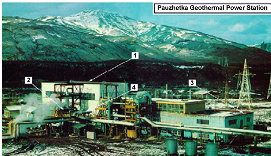
Fig. 15.2 Pauzhetka flash-steam power plant. Key: 1 = power house; 2 = steam inlet pipe; 3 = offices and laboratory; 4 = geofluid inlet. Photo from O.A. Povarov [4] [WWW].
