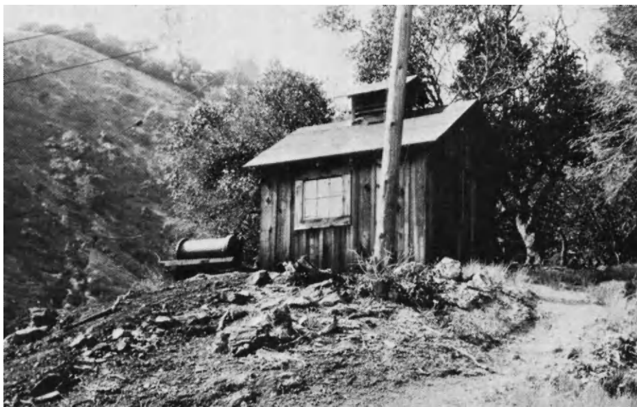
Fig. 12.4 The first power house at The Geysers. It was built about 80 feet east of the No. 1 and 2 wells, and used their steam to produce 35 kW. Photo courtesy of Geothermal Resources Council, pub. in [1].
