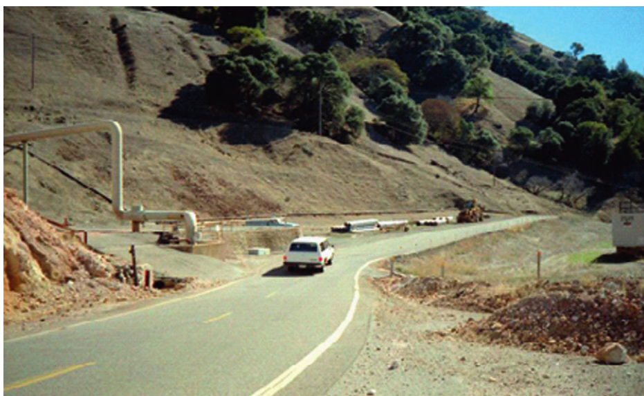
Fig. 12.11 Site of original Units 1 and 2 after demolition and prior to drilling of well GDC-31. The power house was on the left and the cooling tower was on the right. Photo by author [WWW].
