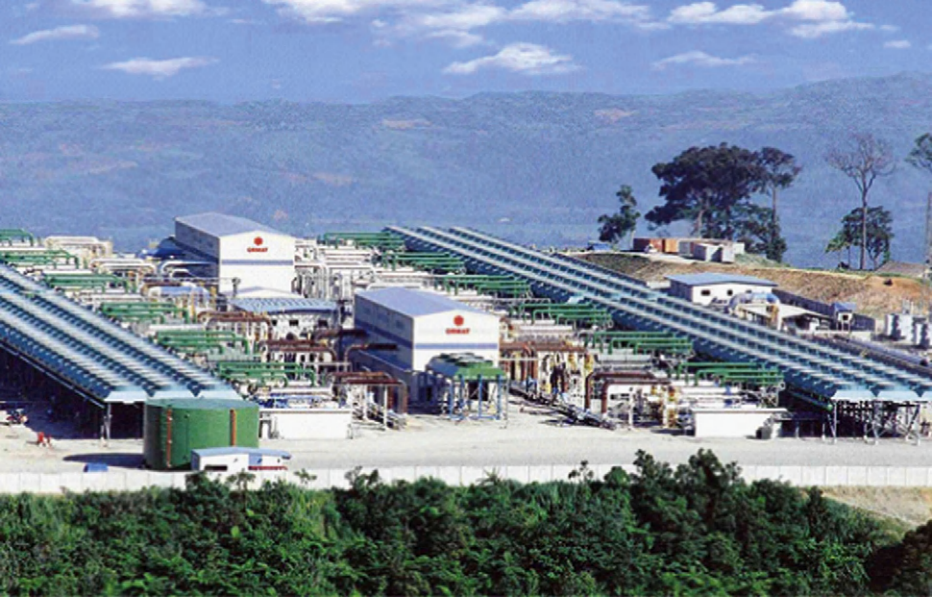
Fig. 9.12 Upper Mahiao integrated flash-binary 125 MW power plant; photo courtesy of Ormat [4] [WWW].
