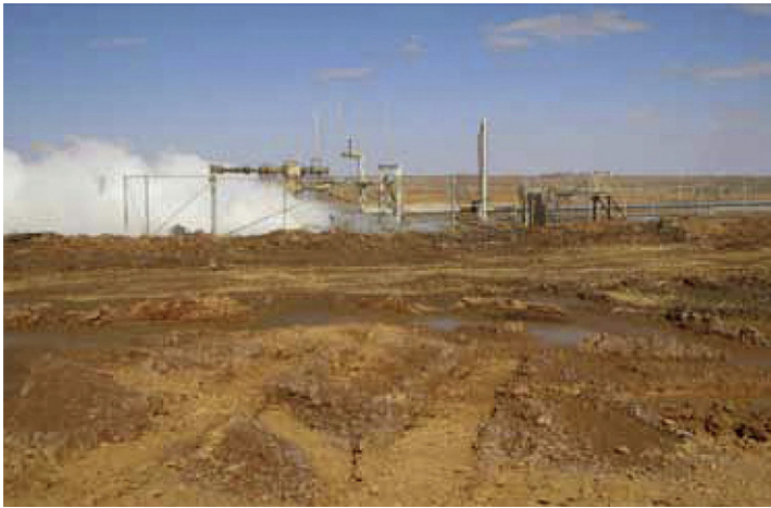
Figure 22.38 Habanero-3 discharging water and steam after blowout on April, 24, 2009; courtesy of Geodynamics Limited [53] [WWW].
