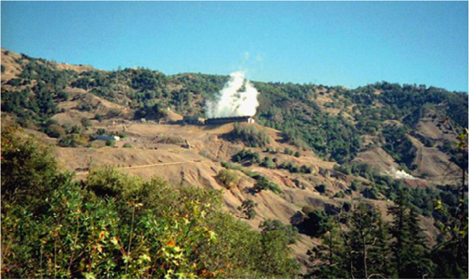
Fig. 12.0 The McCabe plant, formerly Units 5 and 6, as seen from Vista Point looking across Big Sulphur Creek. This is one of 23 power plants that have been built in the rugged Mayacamas Mountains in Northern California. Photo by author [WWW].
