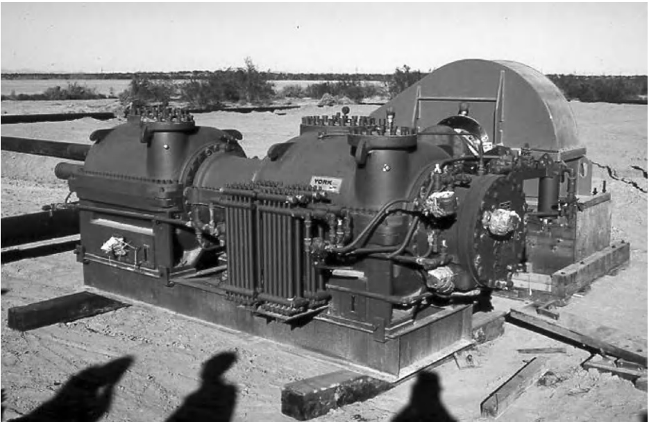
Fig. 18.5 Original turbine awaiting installation at East Mesa. The reduction gear is behind the turbine. March 1978, photo by author [WWW].
