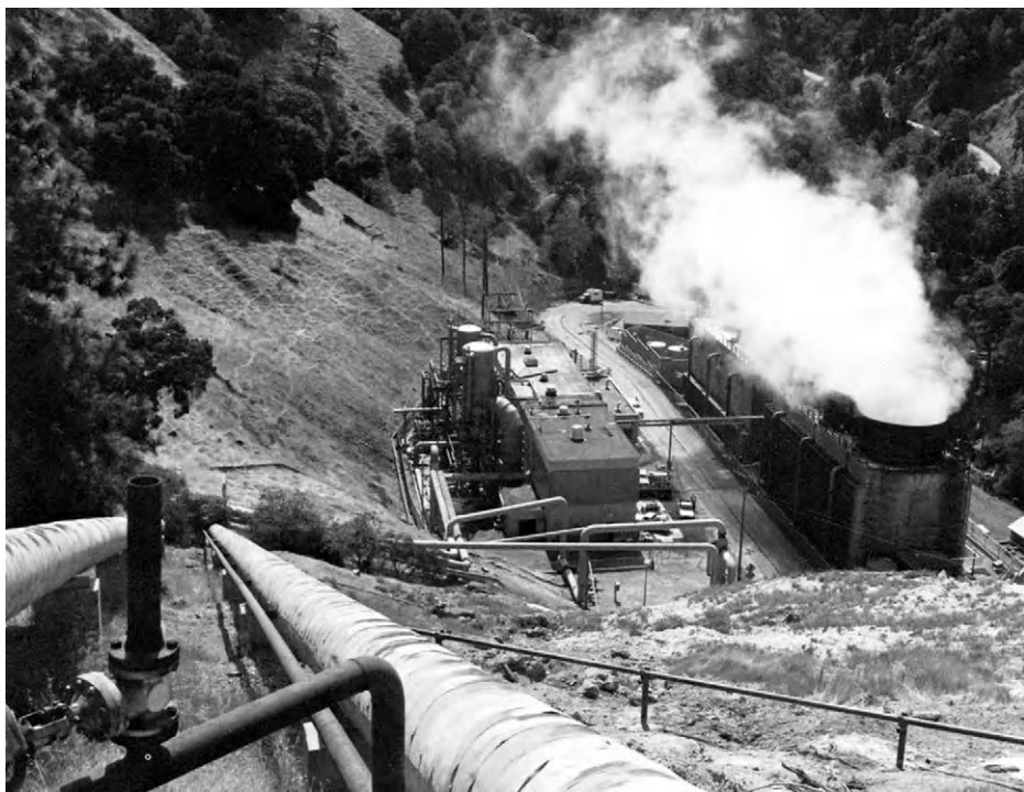
Fig. 12.10 Historic photo of PG&E Geysers Units 1 and 2 looking generally east; Unit 1 is at the rear. The access road ran between the cooling tower and the power house. Big Sulphur Creek lies to the right of the plant, parallel to the main axis of the cooling tower. Note the steep terrain, approaching 45^\circ behind the plant. Photo from [10].
