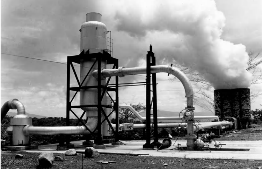
Fig. 5.7 Wellhead separator system at Ahuachapán, El Salvador. Photo by author [2] [WWW].
