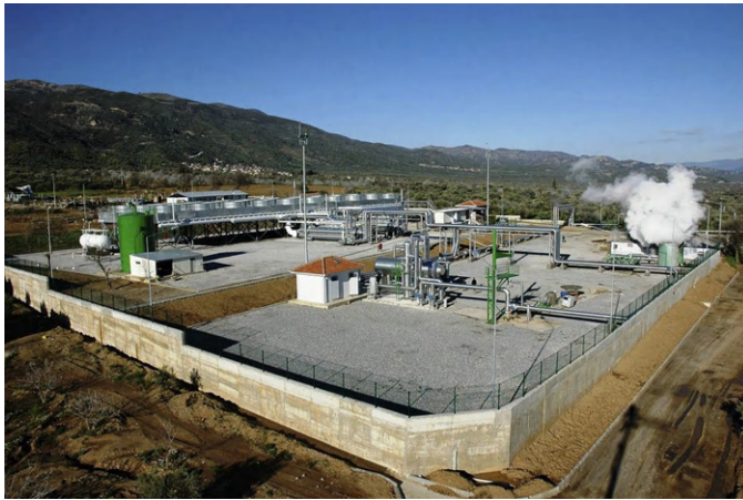
Fig. 21.12 Salavatlı Dora I power plant [16], before construction of Linde Gaz plant. Reinjection well AS-2 is in the front [WWW].
