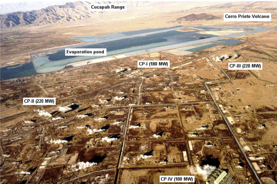
Fig. 13.3 An overview of part of the well field supporting four Cerro Prieto power stations. Photo courtesy of Luis Gutierrez Negrin, CFE [WWWW].
