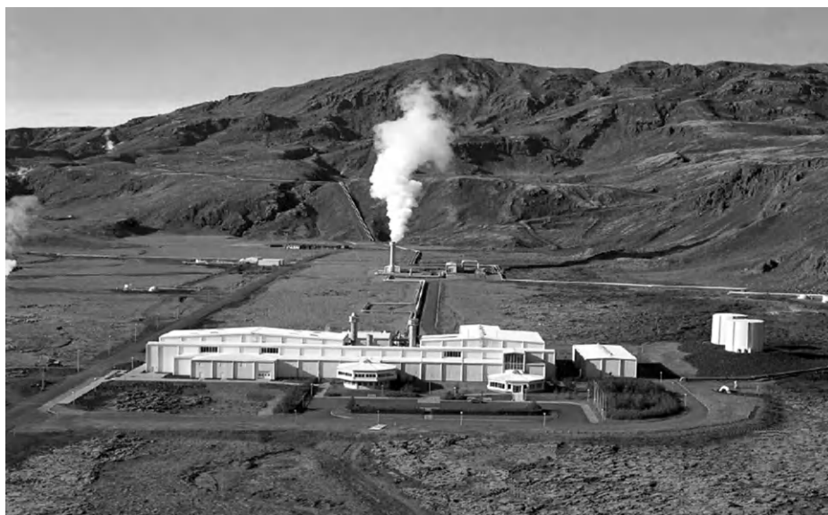
Nesjavellir 60 MWe and 200 MWt geothermal plant, Iceland.
