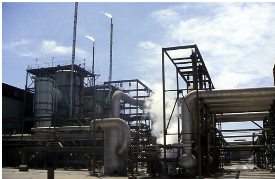
Fig. 13.8 CP-I separated steam arrives through the pipelines from the right, enters the steam header, and passes through the moisture remover prior to being admitted to the turbine. Note the barometric condensers at the rear left and the two tall stacks that are discharging the noncondensable gases along with a small amount of steam. Photo by author [WWW].
