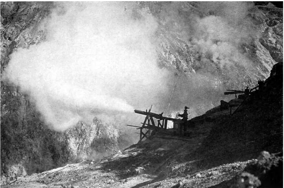
Fig. 12.3 J.D. Grant's first two successful wells at The Geysers. No. 2 is blowing across Geyser Canyon; No. 1 is 40 feet farther up the canyon rim. From Allen and Day [2].
