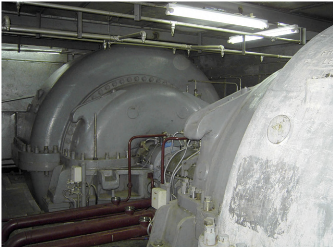
Fig. 21.7 Turbocompressors at Kızıldere Unit 1; photo by author April 2005 [WWW].
