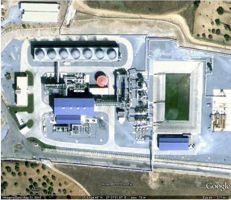
Fig. 21.21 Aerial view of Germencik plant layout, Google Earth, Aug. 21, 2010. The pipeline at the bottom foreground is the brine reinjection line carrying the fluid to the left [WWW].
