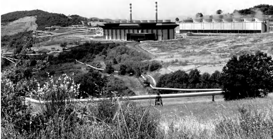
Fig. 11.0 Valle Secolo geothermal power plant, Larderello, Italy; photo courtesy of Enel GreenPower.
