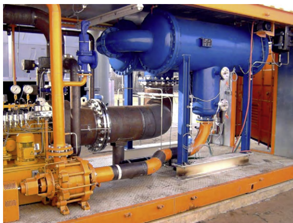
Figure 22.33 Neustadt-Glewe skid-mounted power unit with new condenser installed in 2004 [41] [WWW].
