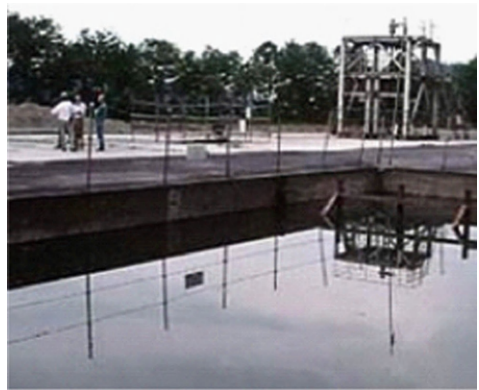
Figure 22.7 Hijiori HDR test facility showing the make-up water holding pond, production well HDR-2a (rear left), production well HDR-3 (center), and separator-silencer station (right) [11].
