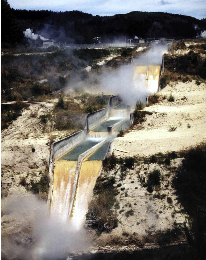
Figure 23.7 Wairakei drop structure (hot-water drainage channel) to the Wairakei Stream not far from the area of maximum subsidence. Photo courtesy of S. Tamanyu, Geological Survey of Japan; photo first published on the cover of Chishitsu News, No. 531, 1998 [WWW].
