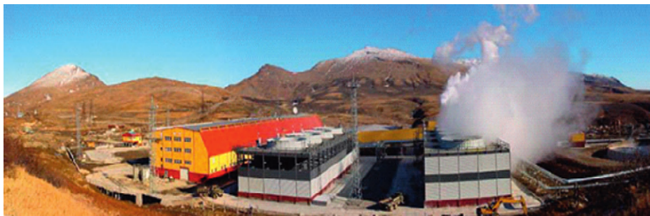
Fig. 15.9 Wide-angle view of the first stage 2 \times 25 MW Mutnovsky flash-steam plant. Power house at left contains turbine-generators and associated equipment to protect them and plant personnel during winter weather. The separator building is out of sight to the left of the power house. Photo from Povarov, et al [8] [WWWW].
