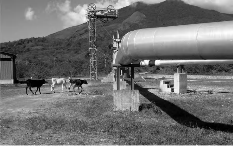
Figure 23.3 Typical pipeline at Miravalles geothermal power plant, Costa Rica. Photo by author [WWW].
