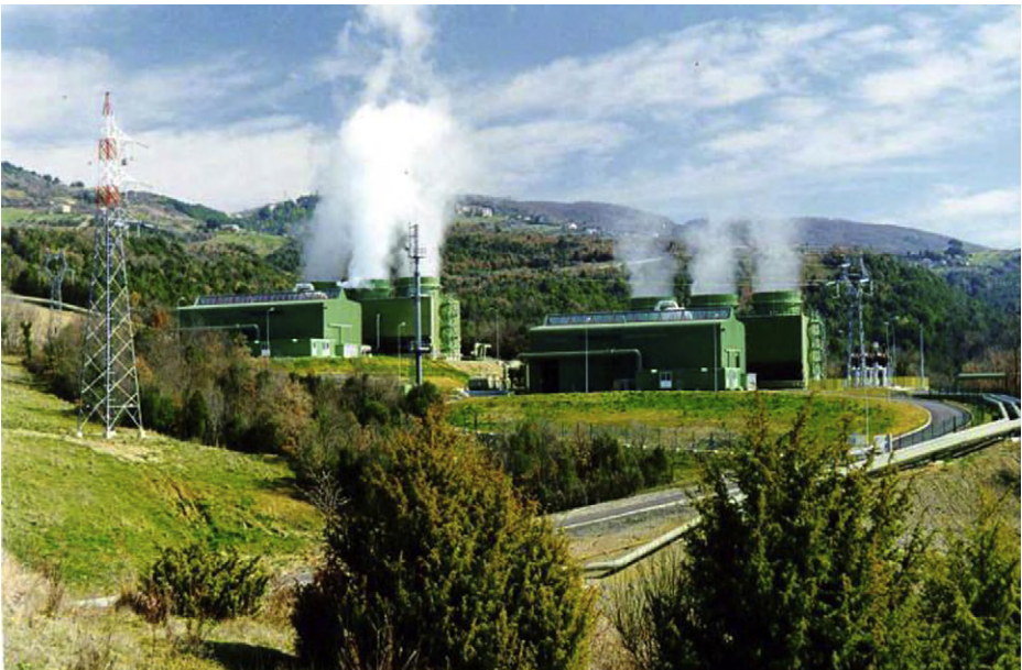
Fig. 11.17 Carboli 2 × 20 MW power units; photo courtesy of Enel GreenPower [WWW].
