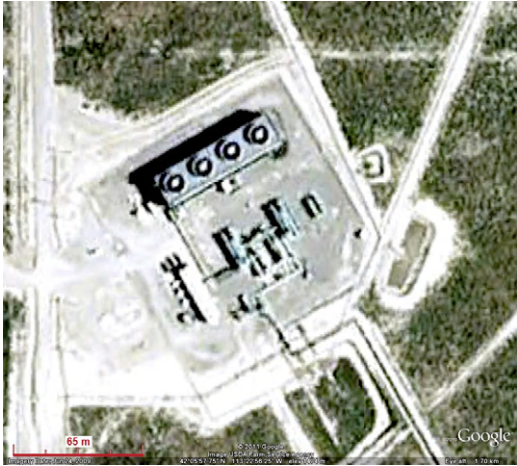
Fig. 20.15 USGeo Raft River, aerial view from Google Earth image, June 24, 2009 [WWW].
